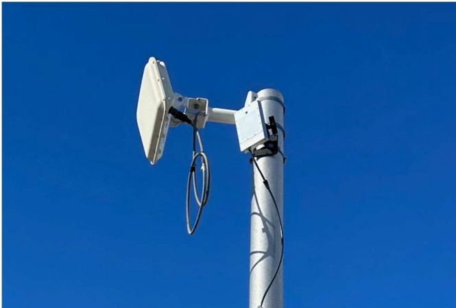
Pilot installation of MegaRadar Fusion Sensor next to existing radar. Existing Side-Fire Radar (left), MegaRadar Fusion Sensor (right)
